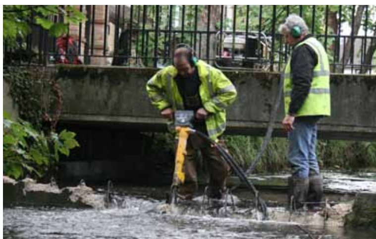
Clockwise from above: fixing faggot bundles in place; planting marginals in the freshly laid gravel; sparks fly as the weir is 'notched', sculpting the river bed; securing the new banks with native plants, breaking down a weir with a pneumatic drill
