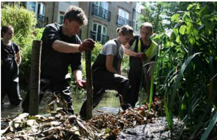
Clockwise from above: fixing faggot bundles in place; planting marginals in the freshly laid gravel; sparks fly as the weir is 'notched', sculpting the river bed; securing the new banks with native plants, breaking down a weir with a pneumatic drill
